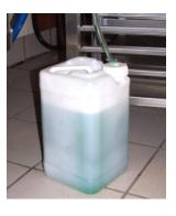
**STEP 3:** Fill the deliming fluid container. Use a non-diluted deliming agent such as Surety™ Delimer or USC Lime-Out. Be sure to read and follow the SDS or safety instructions on the bottle of your deliming agent.
