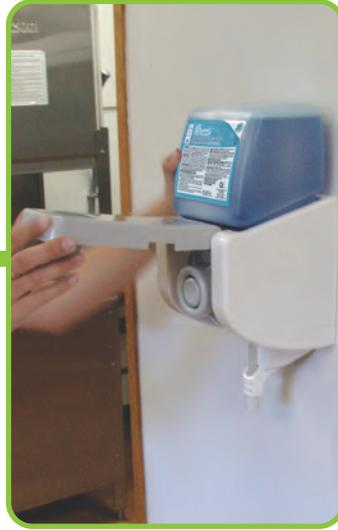
Lift paddle, remove old canister. Properly insert new canister with label facing out into plastic dispensing mount. Move paddle down (canister is locked).
